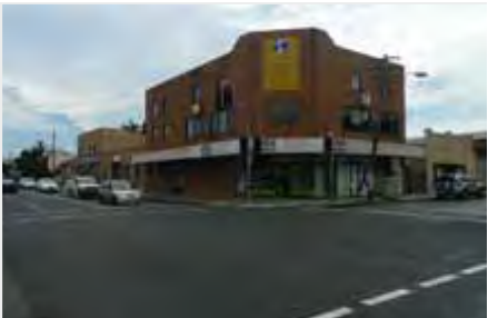
2 Corner Victoria and Sydenham Roads
